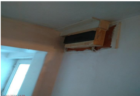
Condition at initial inspection
