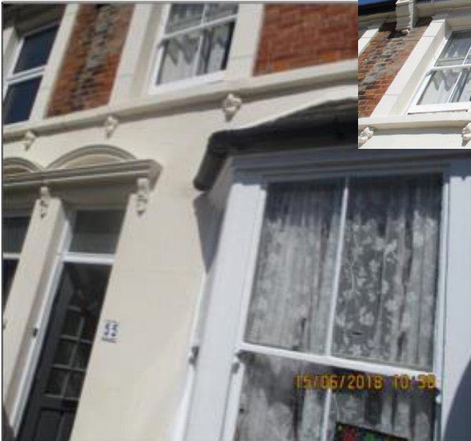
Front elevation after work (above and left)
