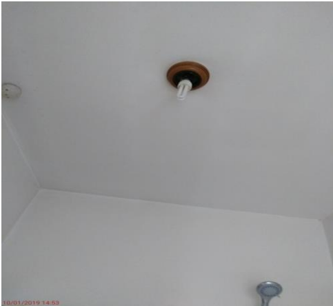
Condition at final inspection
