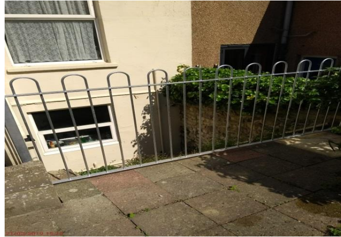
Condition at final inspection
