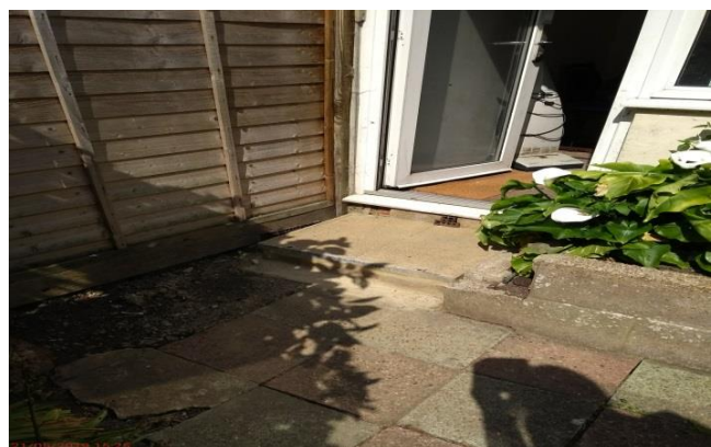
Condition at final inspection
