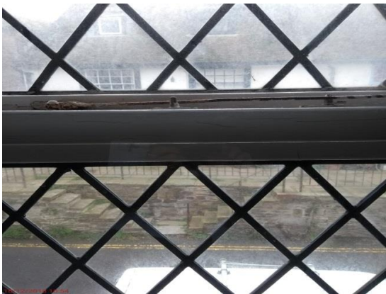
Condition of bedroom window at initial inspection (below)
